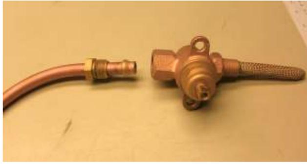
Bill Pancake took the three photos shown above. These photos are of a new valve and outlet nut and feral. The nut has non-standard 9/16 – 20 threads. According to Bill, at one time this nut and feral could be purchased at the local hardware store, but they are now difficult if not impossible to find.
