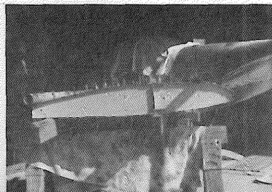
End view (below) of Lyle's method of using two lengths of tubing for eyeball alignment of wing, no twist
